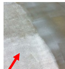
Structured surface (coarse „orange skin“) after the tackifier has been applied with a coarse-pored foam roller and dried off completely.
